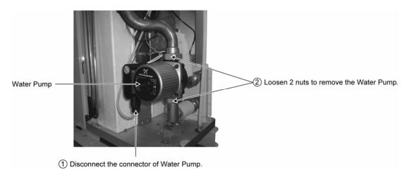
$\triangle$  When reinstall the water pipe, use grease or water at the joining.
